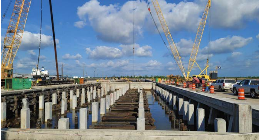
At the Port of Lake Charles in Louisiana, a $30 million rehabilitation project is underway to replace the 1920-era berth structure that's supported by wood pilings and lacks the weight capacity for modern cargo handling.
