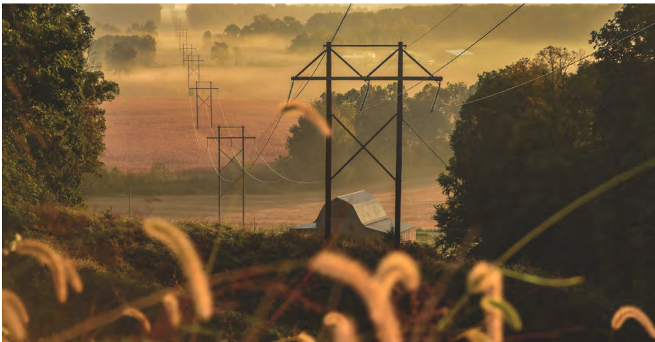
Photo: Hoosier Energy
