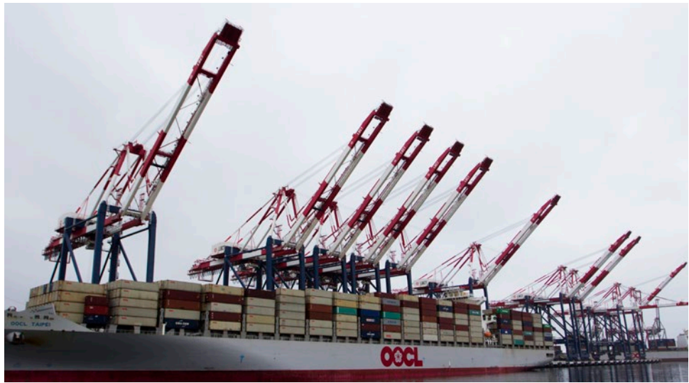
Automated terminals have to accommodate larger vessels, processing massive data volumes and connecting with a growing number of supply chain stakeholders to enable smooth and efficient port operations.
