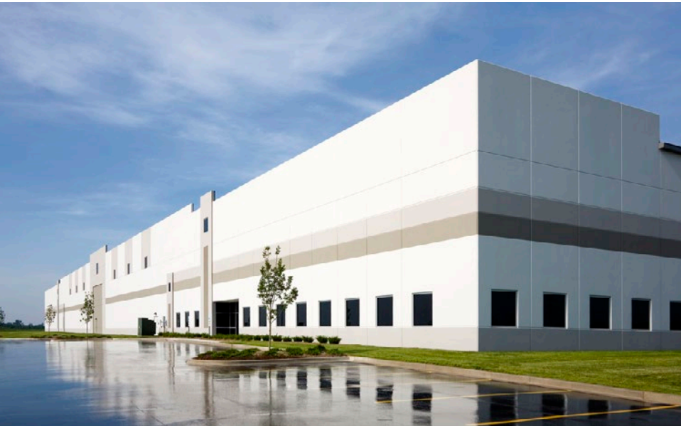
This Panattoni Development building within the Lakeview Commerce Center in Edwardsville, Ill., is composed of concrete tilt-up panels and is designed to expand up to 1 million square feet. This type of new construction helps attract businesses to the St. Louis region.
