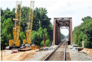
This through-truss bridge over South Carolina's Congaree River had to be replaced to allow clearance for the wide steam generator.
