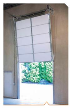
The Kelley Rapid Install system from Entrematic, a provider of warehouse solutions, allows for faster install of loading dock doors to minimize downtime. The system enables dock doors to be installed by one person, and is available on all Kelley steel sectional doors with standard 2-inch or heavy-duty 3-inch tracks.
